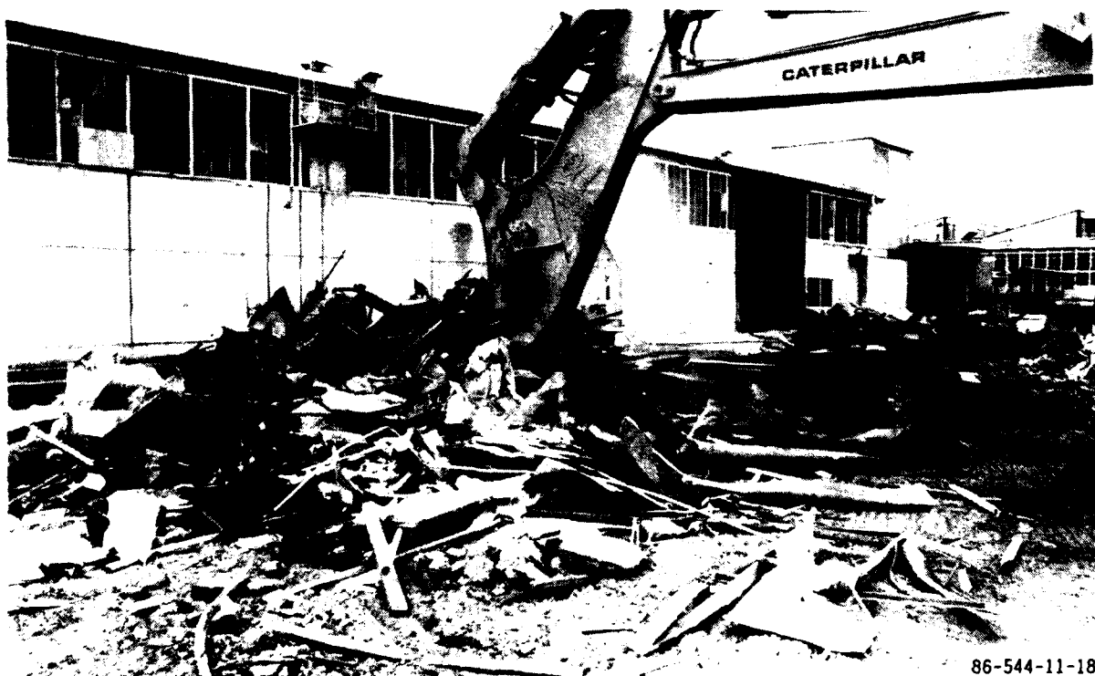
Figure 42. Sectioning miscellaneous tanks and other hardware outside the building.
