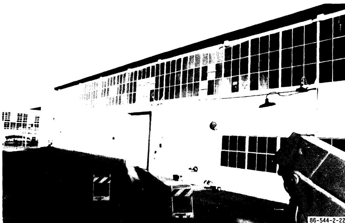
Figure 23. South side of Building 666 showing boarded-up broken windows, closed windows, and closed doors.
