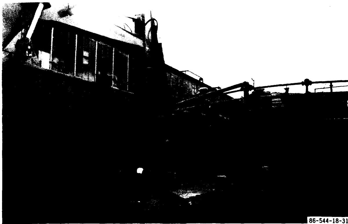
Figure 66. Mechanically shearing the IWTP No. 4 components using the Caterpillar 235/shear.
