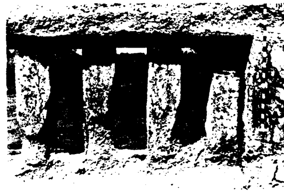
Fig. A.2.9.5.a—Scaling (very severe)
