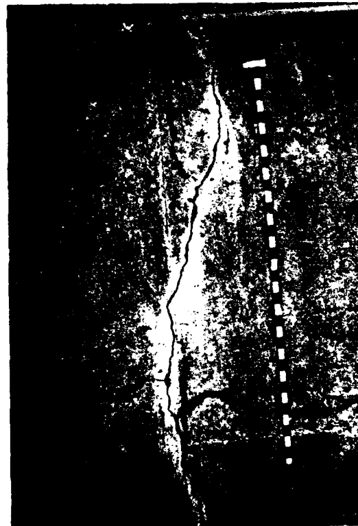
Fig. A.1.1.e—Vertical crack (wide)
