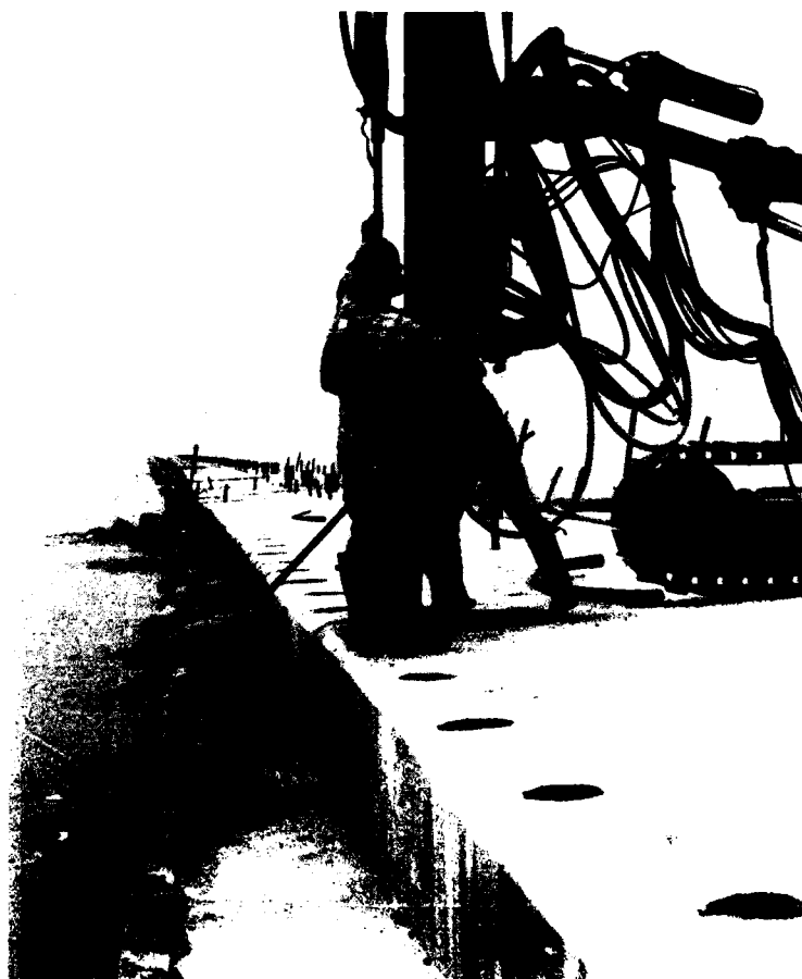
Figure 25. Drilling for rehabilitation sealing of Milwaukee, WI, north detached breakwater
