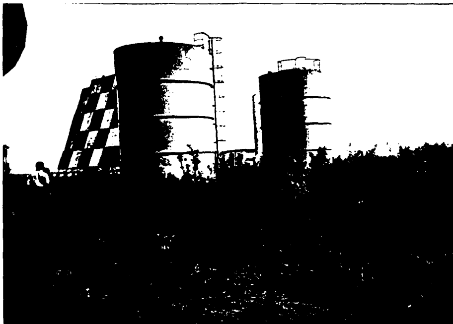
Photo 4. Fuel tanks at Kalakaket Creek RRS, Alaska.
