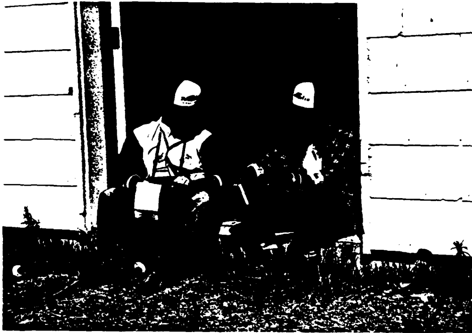
Photo 11. PCB soil testing outside the transformer room.
