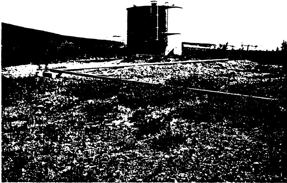
Photo 7. Fuel storage tank and associated piping east of the runway viewed east.
