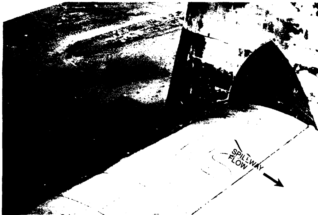
Photo No. 2-21. Spillway Gate in Lowered Position (view from spillway bridge, with reservoir to left).
