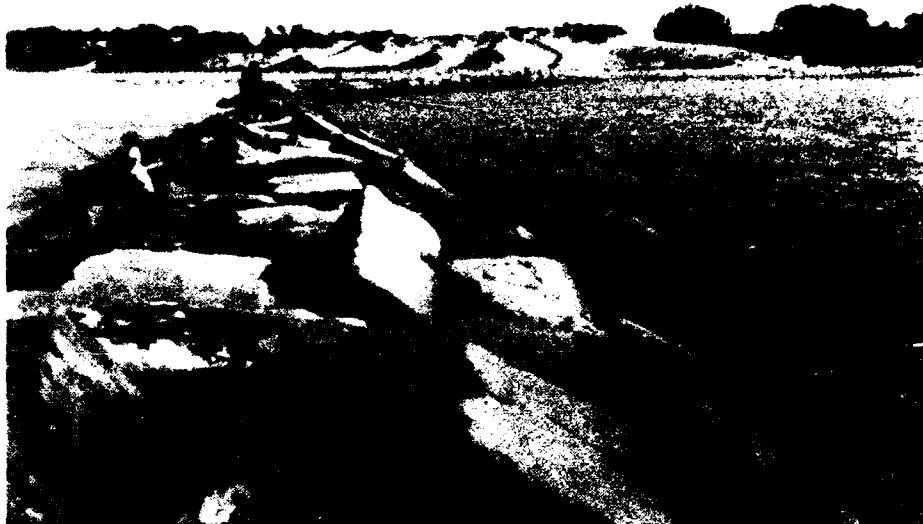
Figure 6. New Buffalo Harbor breakwater constructed with one layer of Bedford Limestone armor stone
