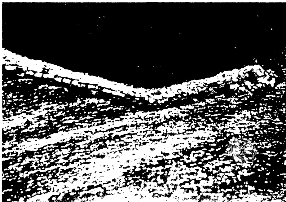
Figure 7. Leland Harbor breakwater constructed with one layer of Bedford Limestone armor stone
