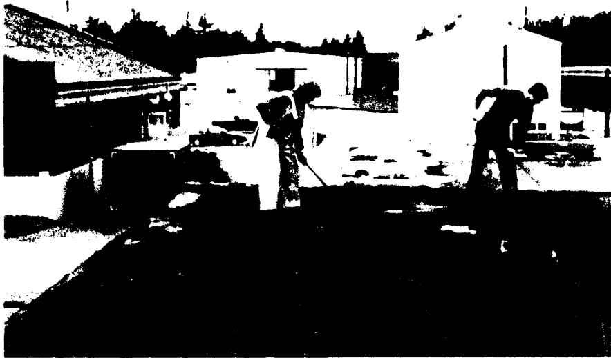
Figure 56. Loose gravel is spudded off the existing BUR.
