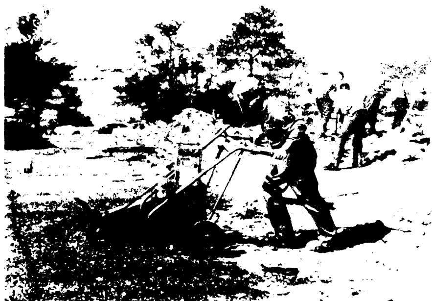
Figure 12. Mechanical cutter being used to separate sections of old BUR.
