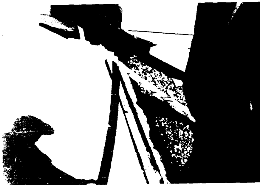
Figure 31. Wood blocking is used to bring an expansion joint to membrane level.
