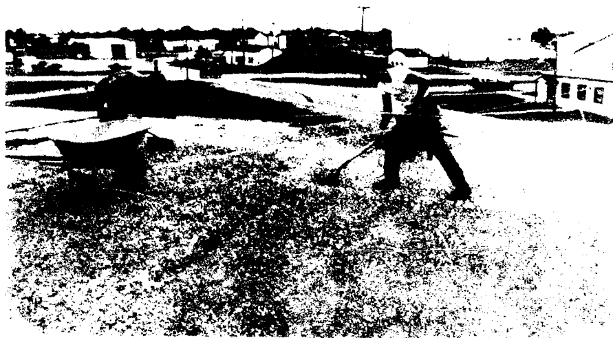
Figure 11. Gravel being removed by shoveling and brooming.
