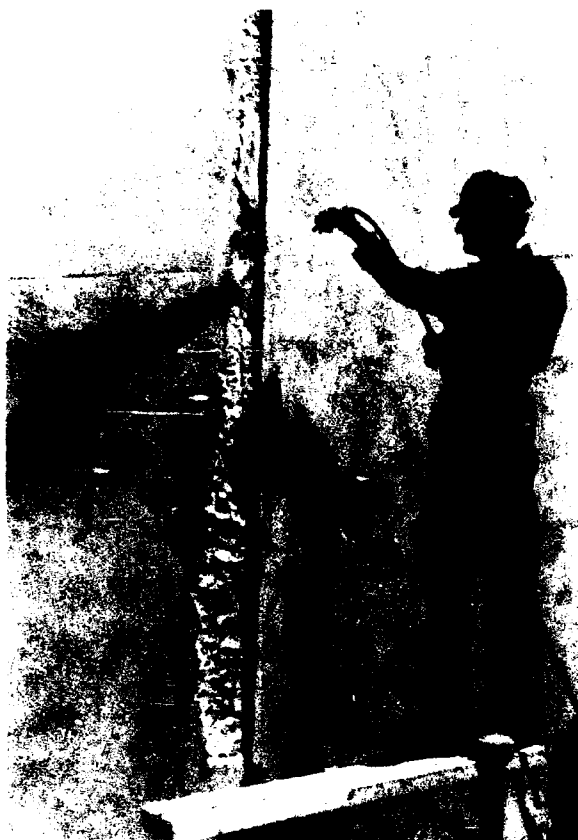
Figure 23. Water and Ali/Cite mixture being applied, Martis Creek Lake Dam
