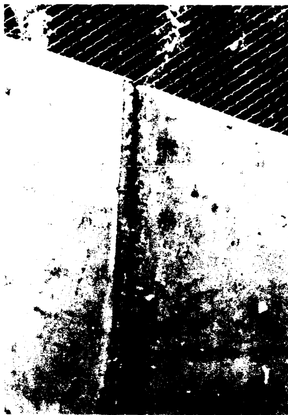
Figure 20. Prepared surface with saw-cut edges, Martis Creek Lake
