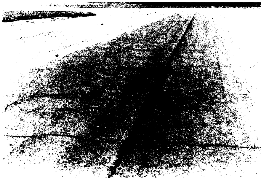
Photo 12. Low severity reflective and block cracking, typical of Taxiways 1 and 3 (T2A1, T2A2, T3A, and T4A)
