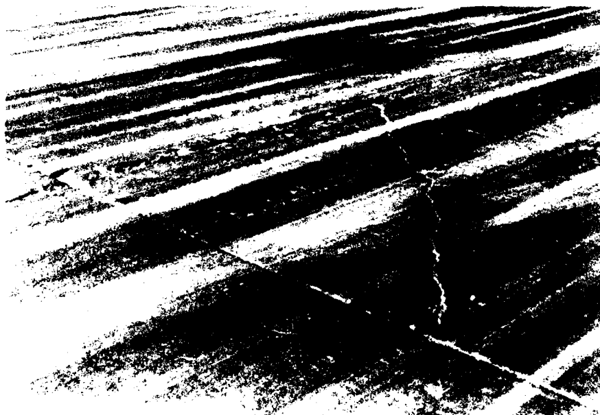
Photo 6. Low severity corner break, Runway 14-32 (R4A)
