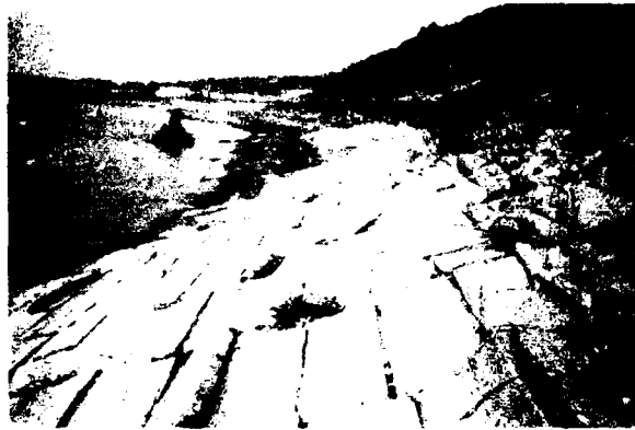
a. Photograph of revetment along the shore
