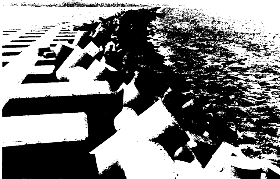
Figure 7. Tribar with toe buttressing stone and concrete rib cap repair section of Hilo Breakwater, Hilo Harbor, Hawaii
