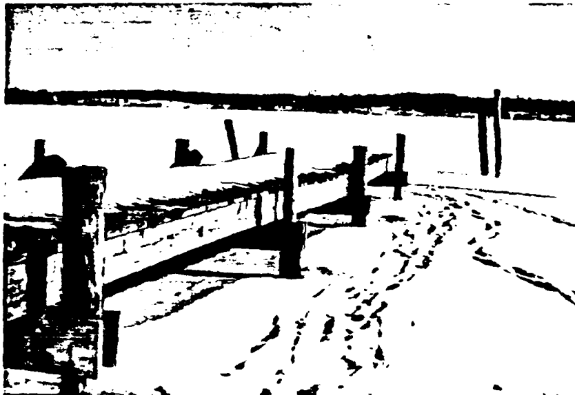
Figure 49. Dark Hole pile dock.
