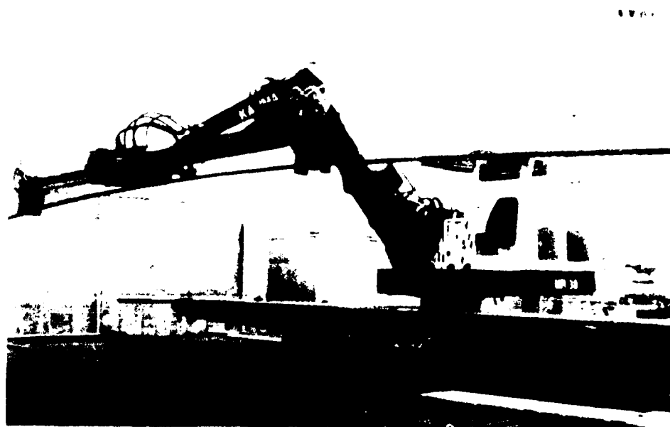
Figure 14. Kajima re-bar-placing robot.
