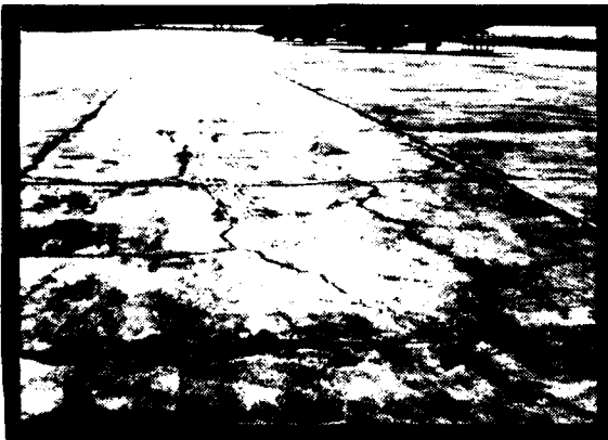
PHOTO 7: Typical shattered slabs concentrated on the apron taxi route. These slabs should be replaced.
