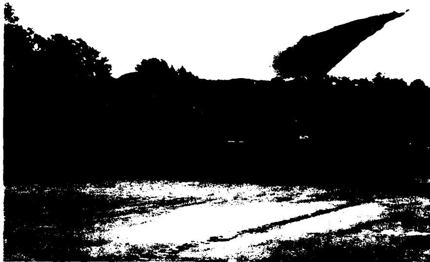
Figure 15. Using an irrigation sprayer to place fine material on Teepeeota Point in August of 1984.
