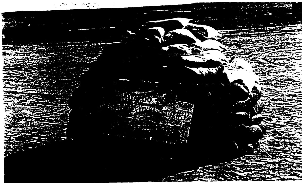
Figure 2. Typical Sandbag Confinement for Steel Drums
