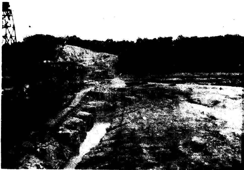
Photo 109 - Power excavation (May 1979)
