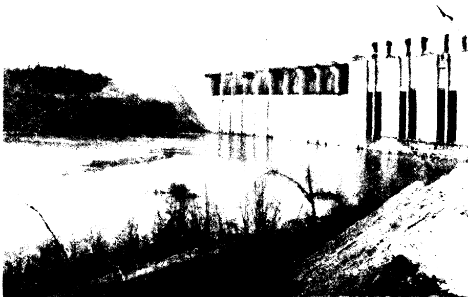
Photo 45 - Upstream side of dam shortly after second stage diversion (January 1982)
