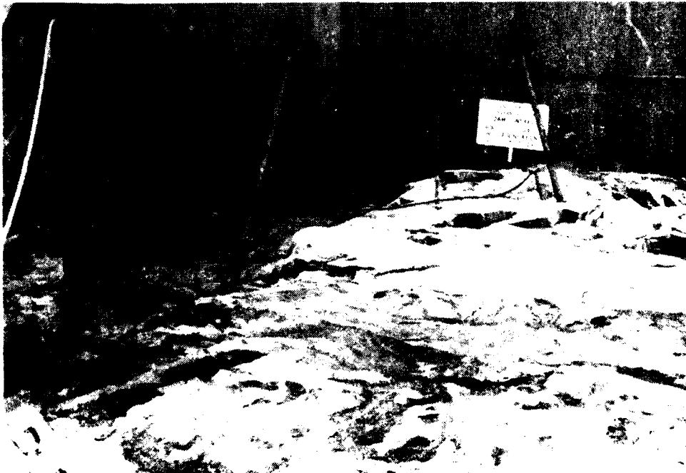
Photo 65 - Monolith 10 foundation (October 1979)
