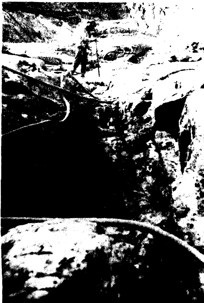
Photo 136 - Foundation conditions, Georgia west - approximately Stations 9+00 to 10+00. Some additional excavation was done in this area.
