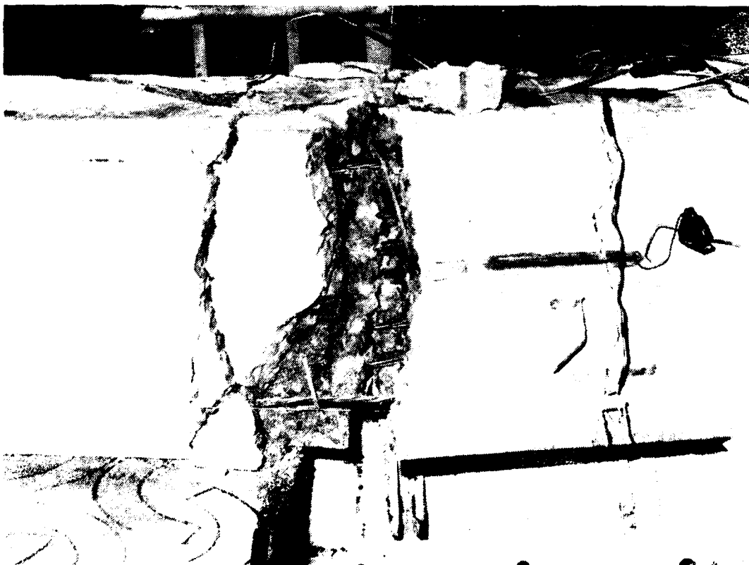
Figure B-168. MK16 tension cracking at failure.
