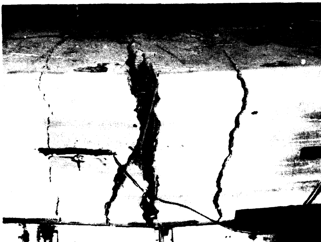
Figure B-216. MK23 tension cracking at failure.
