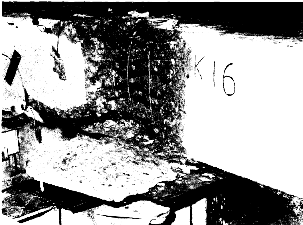
Figure B-167. MK16 compression spalling at failure.
