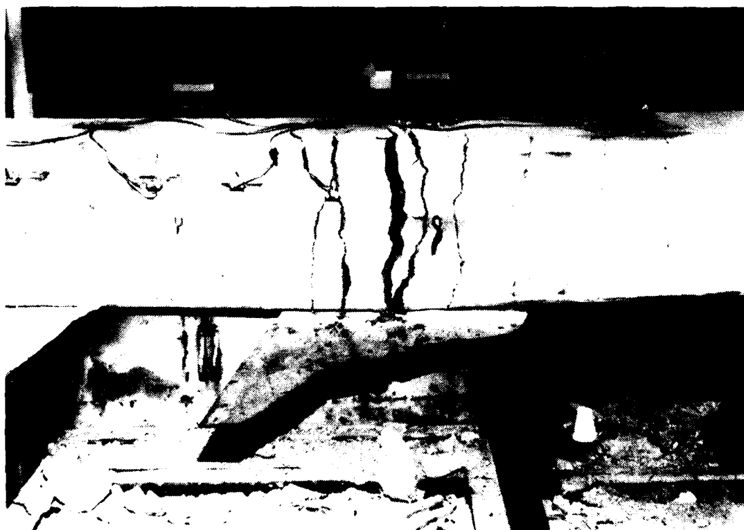
Figure B-232. MK5A tension cracks at failure.
