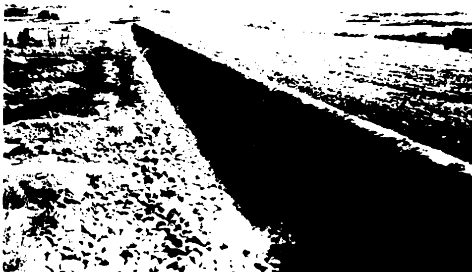
Figure 55. Historic view (1937) of Dam 357 spillway showing the stone masonry weir wall and apron.
