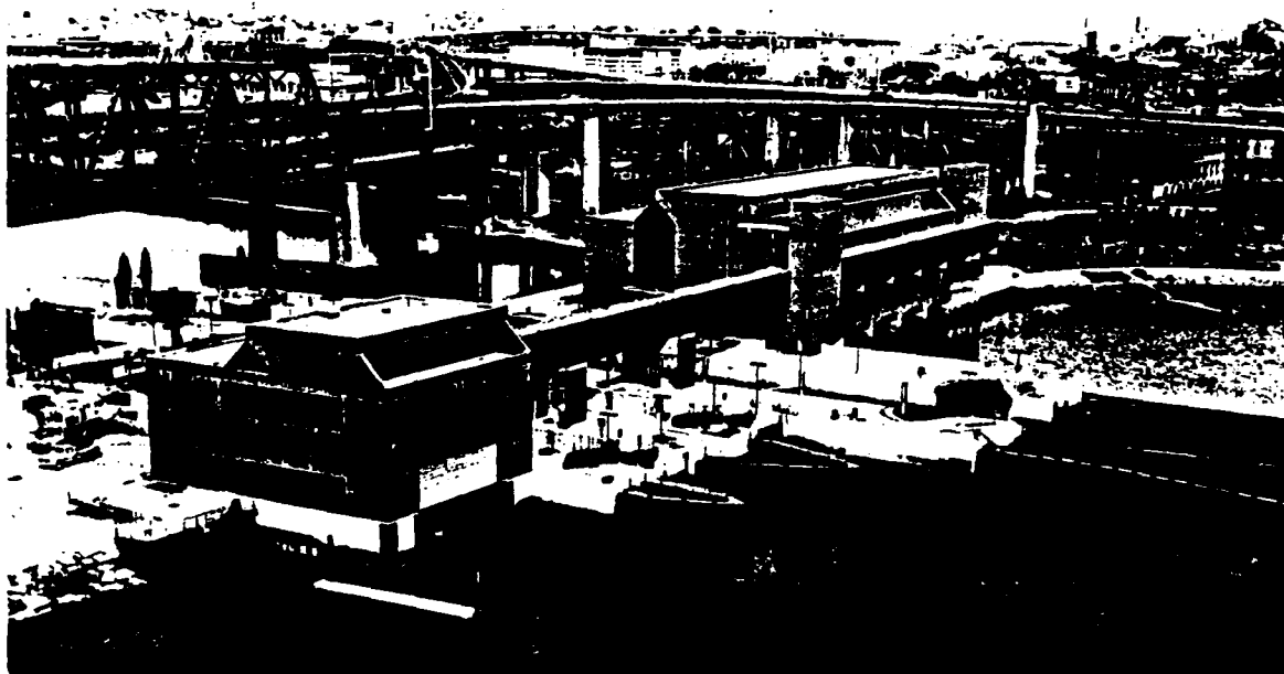
CHARLES RIVER DAM PROJECT - Completed by the Corps of Engineers in 1978 at a cost of $59 million, located between Charlestown and Boston's North End. The project includes a fishway, a pumping station and three navigation locks across 440 feet of the Charles River and 350 feet of earthfill dam across the rest of the river. To harmonize the project with the historic environment of the communities it protects, the structural design features a facade of red water-struct brick traditional to Boston. The new Paul Revere Landing Park on the Charlestown abutment commemorates the Patriots midnight ride. The preservation of 8500 acres of wetlands as part of the Natural Valley Storage component of the project received several environmental awards. The Metropolitan District Commission operates and maintains the dam.
