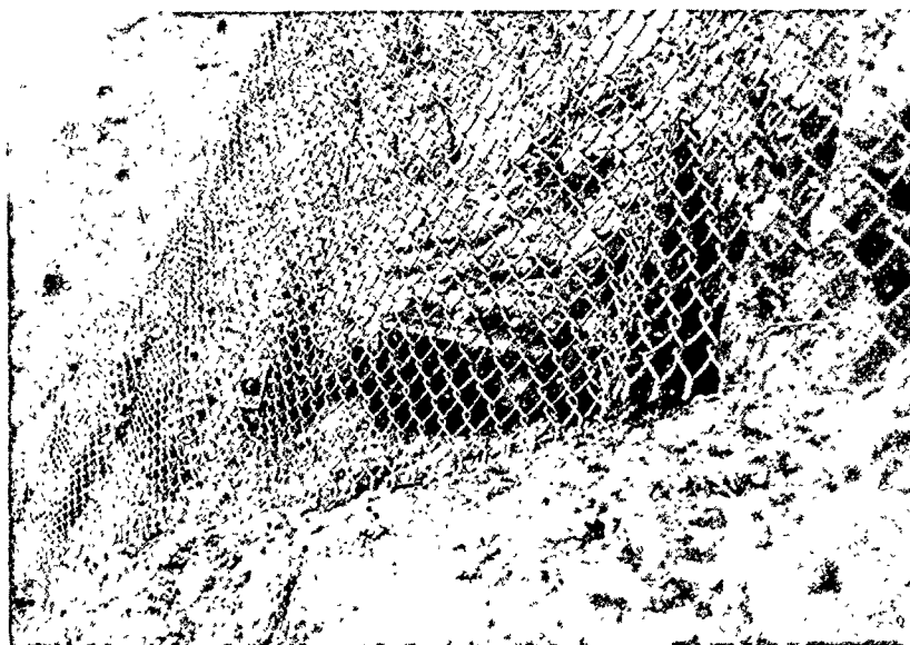
PHOTO 27. Rock bolts and protective wire mesh, Feb 64
