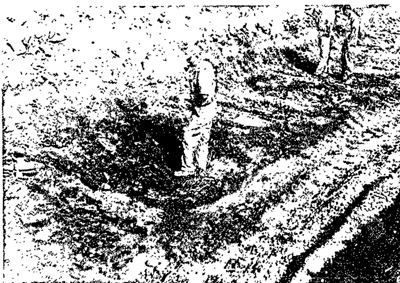
PHOTO 11. Upturned Eagle Ford shale on the down-thrown side of the South Fault in the upstream fault excavation.
