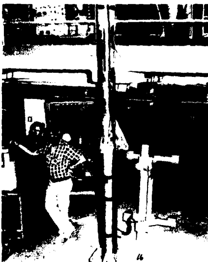
Missile Suspended from Elastic Cords Body Bending Tests (fig. 16)
