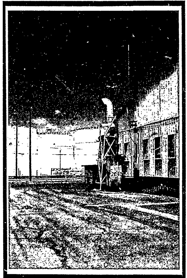
21. VIEW OF EXHAUST VENT AND SHED
