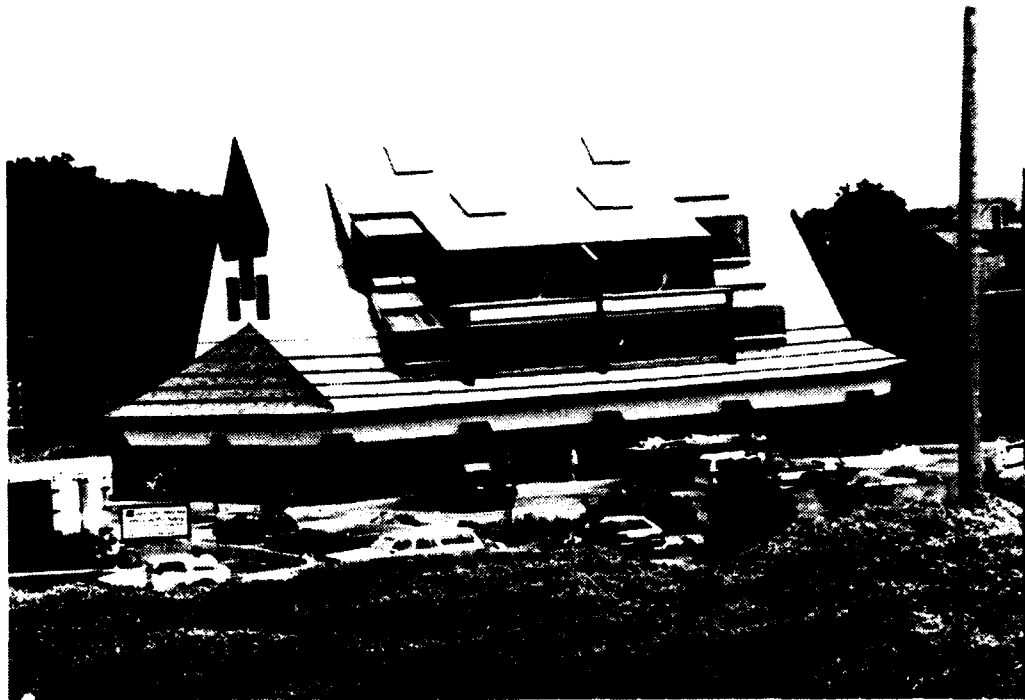
Figure 5. South View of Completed United Federal Bank
