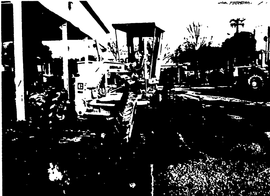
Figure 2.19 Grader Windrowing Wet Mixed Material
