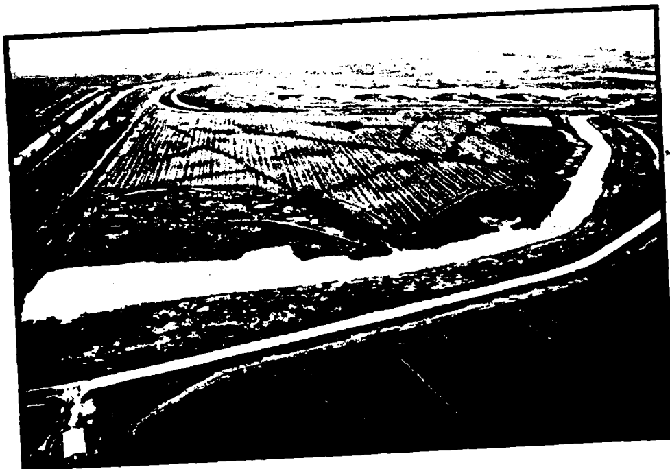
Landfill No. 2 (FACING SOUTH)
