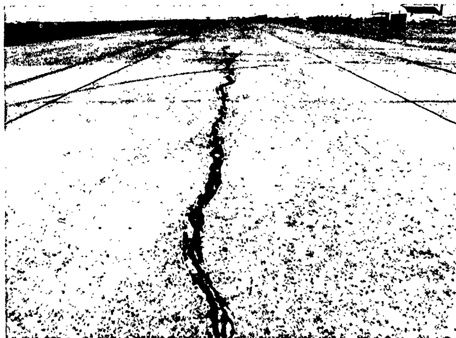
Photo 18. Sealed longitudinal/transverse crack on T3A
