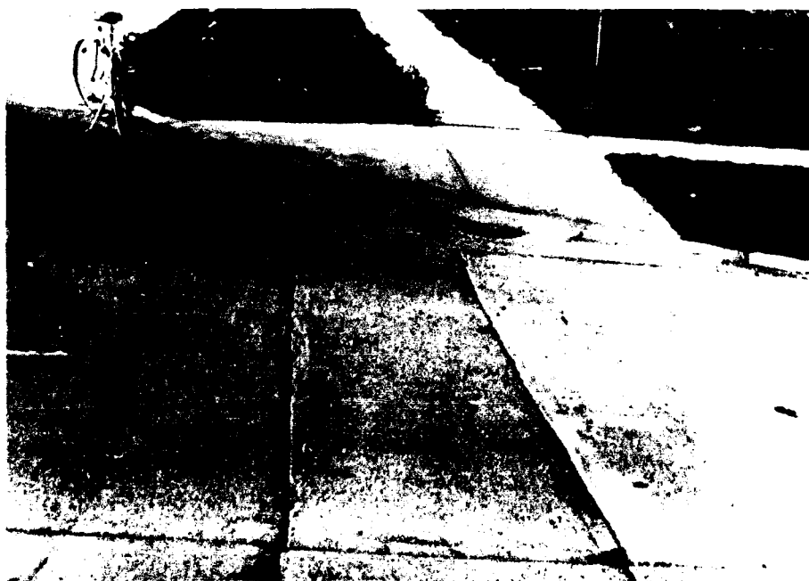
Figure A81. Examples of low-severity patching (large, utility cuts).
