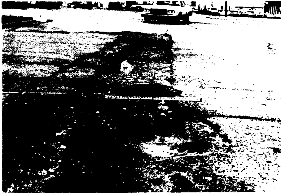
Figure A34. High-severity utility cut patching.
