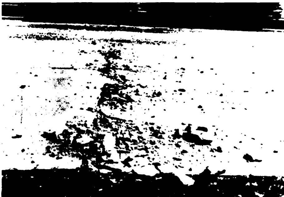
Figure A57. Examples of medium-severity blowup/buckling.
