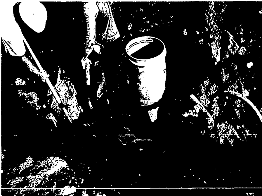
98. Blue Springs Lake, 12 August 1985, Neg. No. 538. Perforated PVC pipe placed in upstream sand drain at station 76+60.
