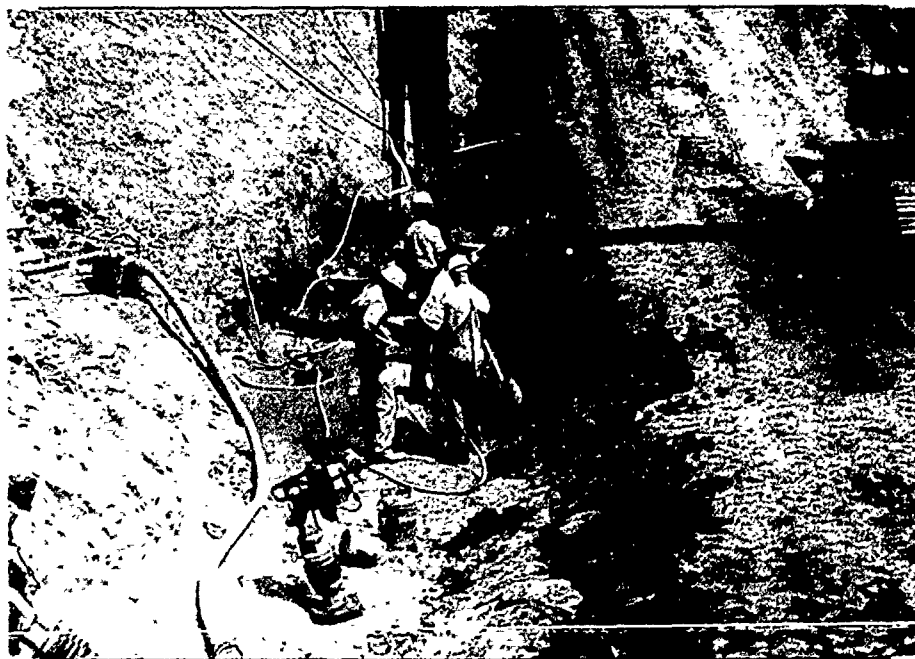
34. Blue Springs Lake, 13 August 1983, Neg. No. 186. Left abutment cutoff trench. Foundation clean up at station 97+10, prior to start of pervious placement.
