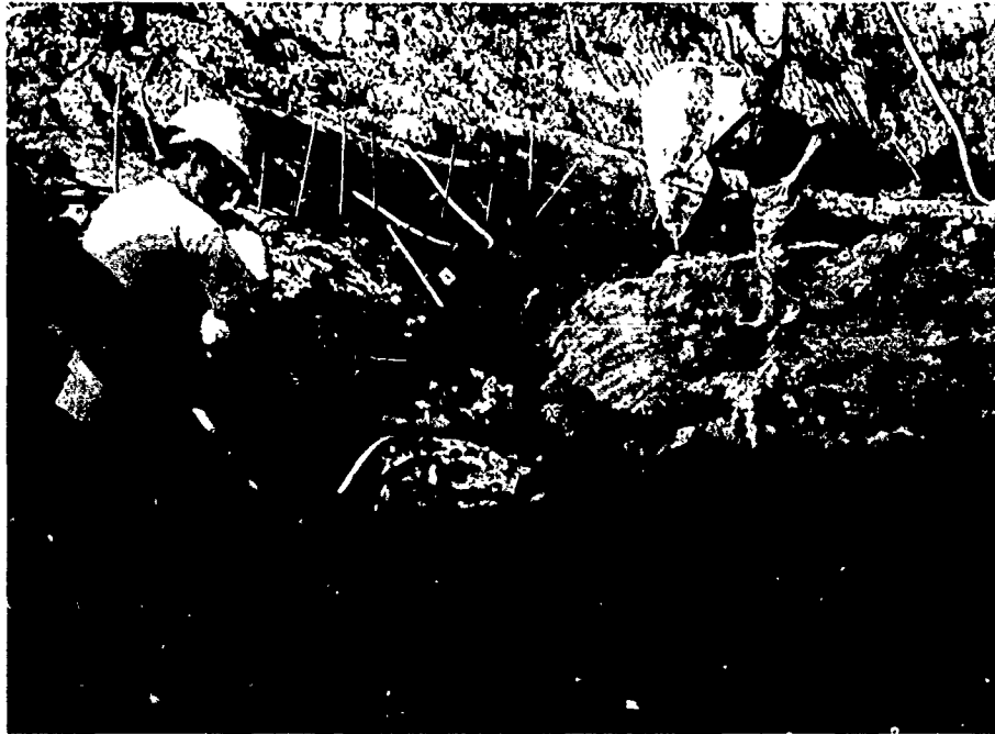
97. Blue Springs Lake, 12 August 1985, Neg. No. 536. Right abutment upstream sand drain at station 76+30.
