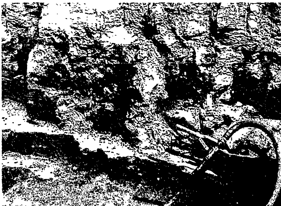
127. Blue Springs Lake, 19 August 1986, Neg. No. 680. Right abutment, cutoff trench at station 74+15. View of downstream wall after open fractures and joints were dry packed. The head of rock-hammer is at El. 802.5 at station 74+20.
