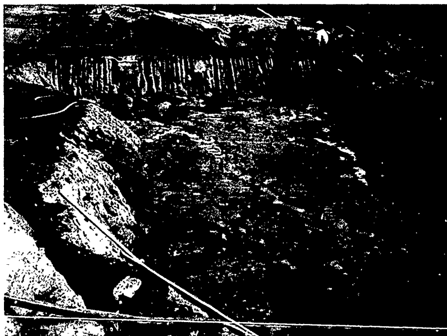
76. Blue Springs Lake, 20 May 1985, Neg. No. 440. Left abutment cutoff trench. From station 98+00 looking downstream. View of floor after cement sand slurry. Note results of line drilling on face of Pleasanton "B" Sandstone.
