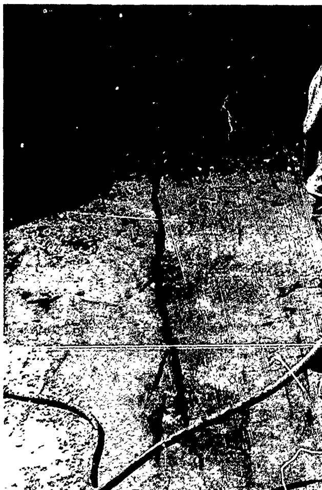
24. Blue springs Lake, 11 July 83, Neg. No. 147. Tower excavation. Open joint in floor bearing surface from station 47+57.1 to station 47+73.4. Looking downstream.
