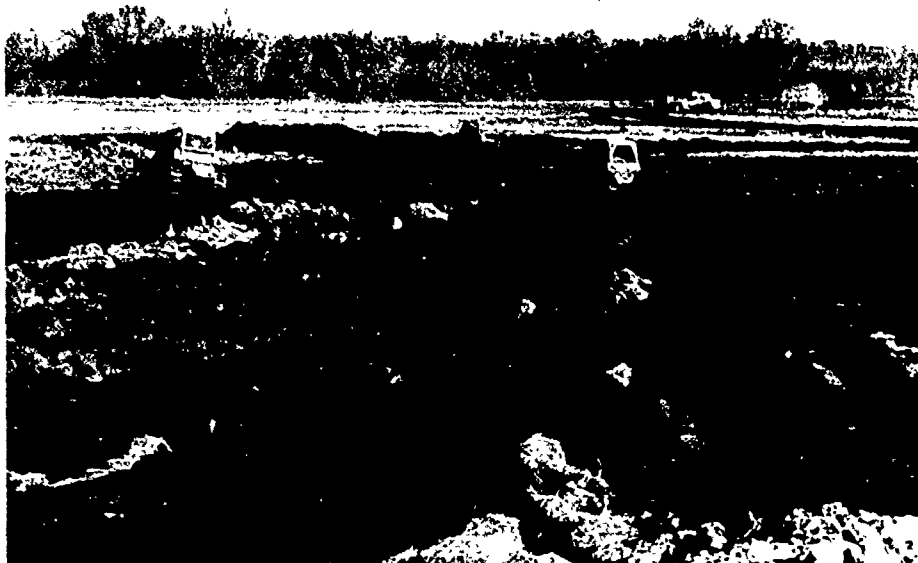
5. Blue Springs Lake, 15 November 1982, Neg. No. 52. Dam foundation at station 92+00. Removing objectionable material, looking north.
