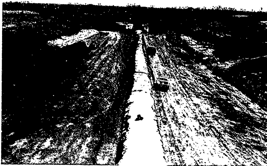
Figure 59. Outlet works looking downstream from tower.
