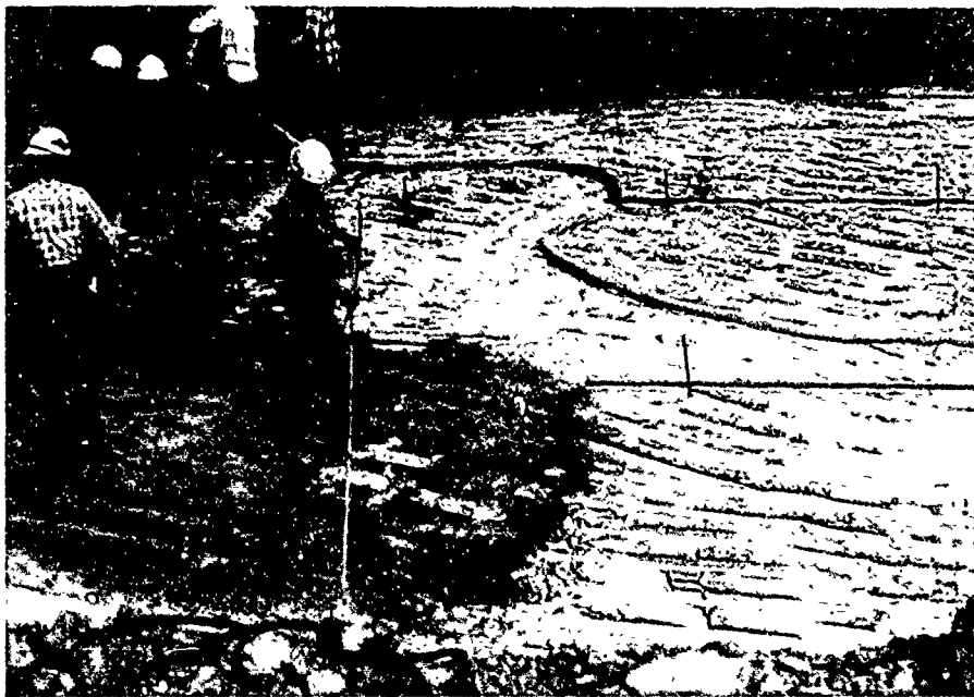
Figure 34. Intake structure foundation - spraying aerospray.
