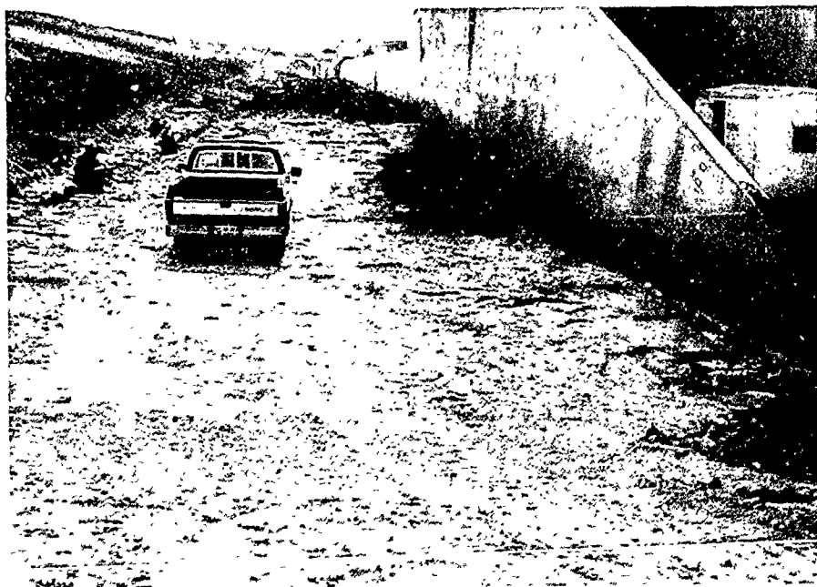
Figure 38. Outlet works, left side looking downstream at intake structure wing walls showing fresh shale surface.
