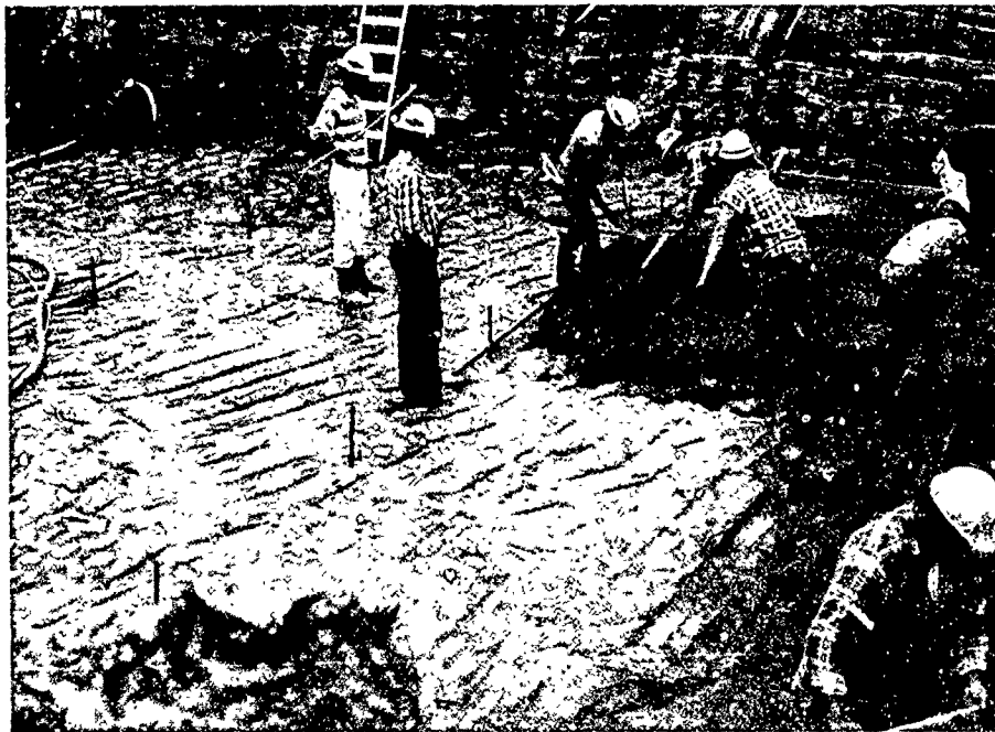
Figure 36. Intake structure foundation - placing protective concrete.
