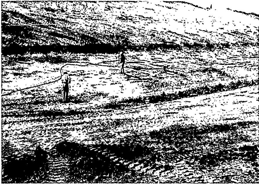
Figure 61. Outlet works, right side, looking downstream. Cleaning shale surface prior to placement of fill.
