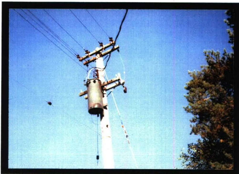
4. LEAKING POLE TRANSFORMER LOCATED NEAR THE GSA BUILDING
