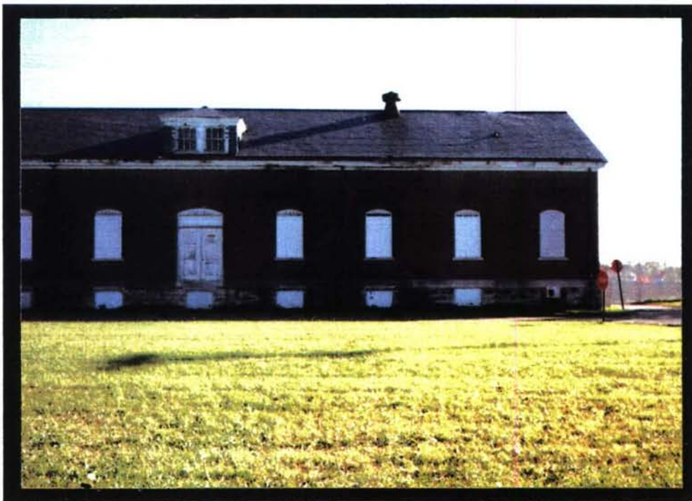
2. BUILDING 138 - VIEWED FROM THE NORTH LOOKING SOUTH
