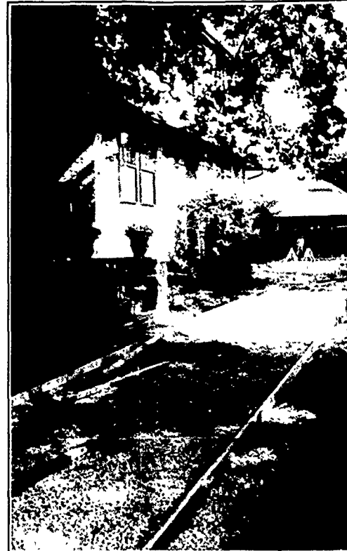
c. New driveway under construction at 112 E. Stewart. Four inches of concrete, reinforced with wire mesh, was poured. The driveway was constructed to replicate those that were damaged. June, 1989.
