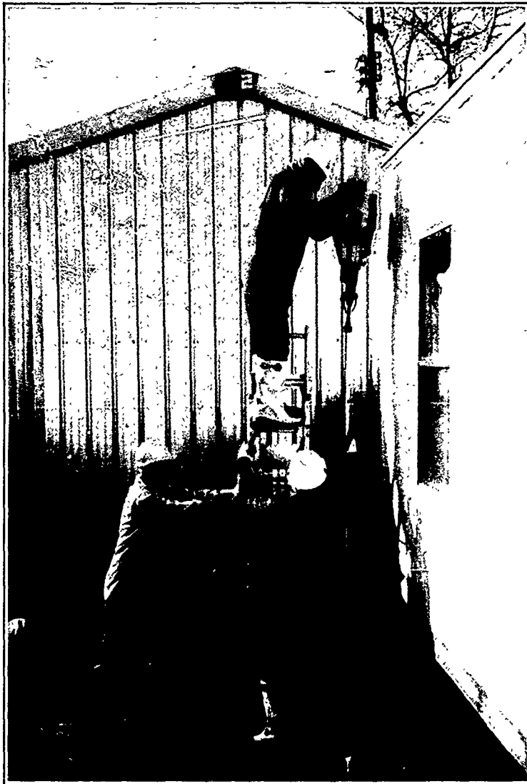
a. Workers driving aluminum conduit tubes in the jobsite administration area. The OSF is in the background; crew trailer is at right. A "Cobra" gasoline powered hammer, manufactured by Atlas-Copco was used to drive the pipe. A steel penetrometer point on the penetrating end of the pipe facilitated penetration and kept soil out of the inside of the pipe. The pipe in this photograph is being driven through the pavement of E. Stratford Avenue, in the vicinity of the sewer lateral from the 105 residence. Subsequent subsurface logging indicated that there had apparently been considerable exfiltration of radioactive contamination from the lateral. This was confirmed when the area was excavated.
