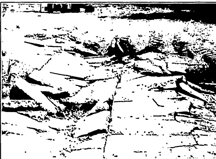
b. Example of damage to the driveways caused by the forklift transporting rad-waste boxes. March, 1989.
