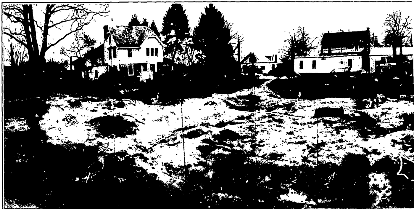
Fig. 7:4 - Jobsite Facing South from the 112 E. Stewart Property Near the End of the Final Phase of Soil Excavation. The photo mosaic is taken from the same perspective as Fig. 7 above. The two garages and the 105 basement are gone, along with approximately 4100 tons of contaminated soil. The irregular excavation grade reflects how the radioactive contamination was distributed in the subsurface. March, 1989.
