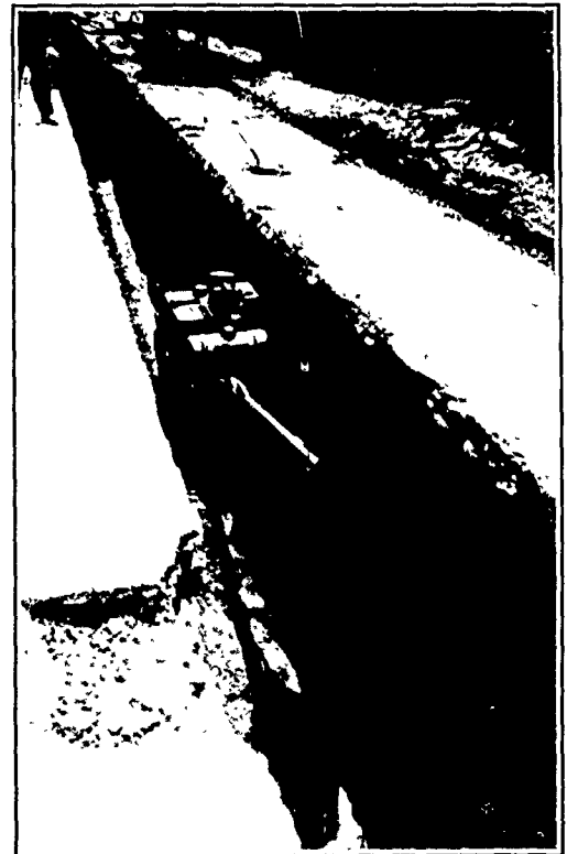
o. Backfill was compacted to 95%-98% maximum dry density.
