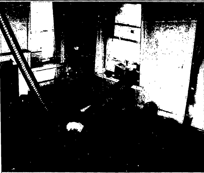
HEPA filtered air was exhausted from rooms on the upper levels of the house. Duct passing through window at right draws filtered air exhausted into the room located on the porch outside the house.
