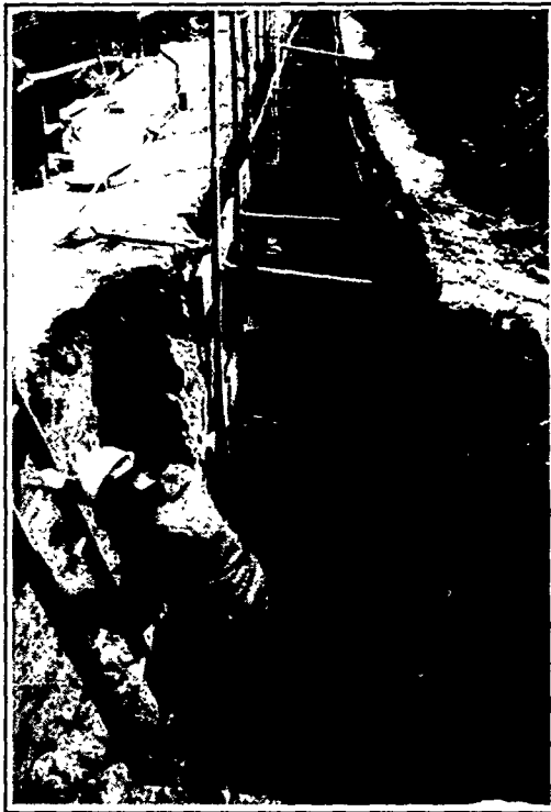
a. 4-foot wide trench was excavated and shored to expose the existing contaminated sewer line (right) and provide space for laying the replacement sewer line beside the existing line (b.). Photo taken facing downstream (east).
