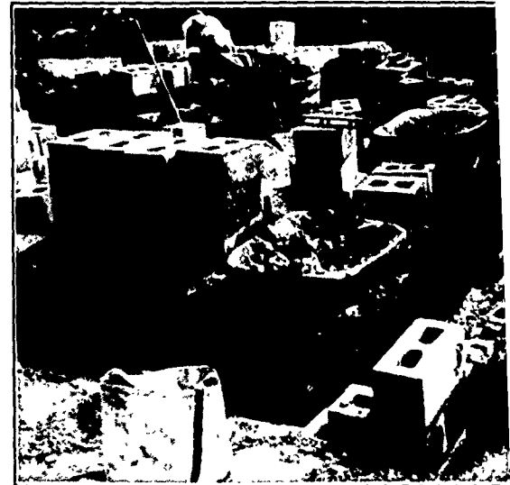
f. The upper part of the foundation consisted of concrete blocks. May, 1989.
