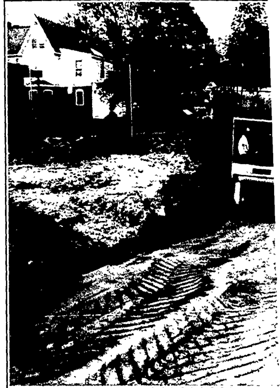
b. Removal of soft clay beneath the new location of the foundation. The excavation was backfilled with sand, compacted in layers. Photo taken facing west, May, 1989.
