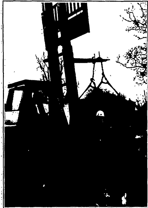
d. Lifting a loaded B-25 box out of the 105 basement packaging containment.
