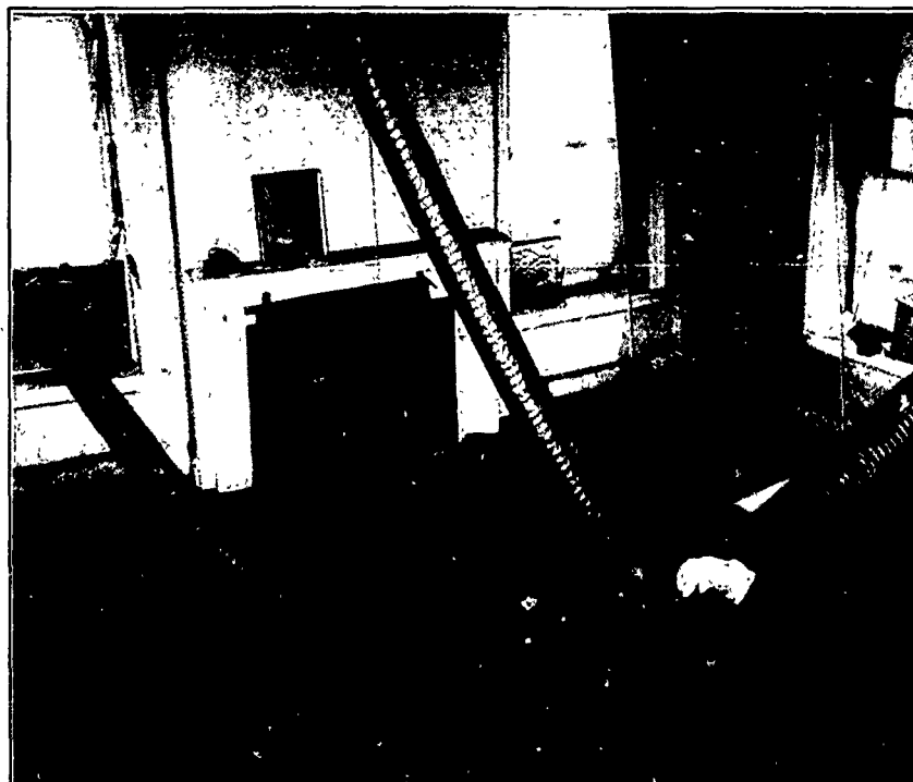
c. First floor living room into which HEPA filtered air was exhausted from rooms on the upper level undergoing interior dismantlement. Duct passing through window at right draws filtered air to the main 2000 cfm HEPA unit located on the porch outside the house.
