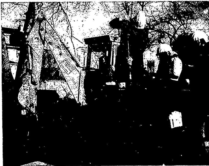
FIGURE B26. Workers Packing Waste Bin with Contaminated Soil
