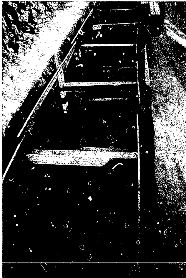
FIGURE 24 Stratford Avenue Sewer Line Replacement with French Drain
