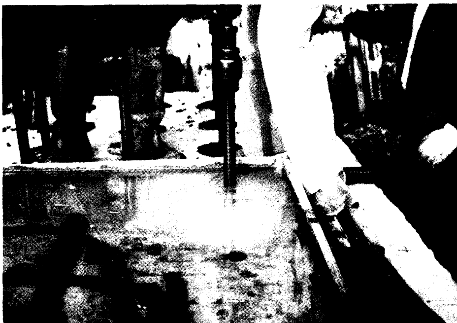
Figure 6. Anchor installed or spun into a submerged hole
