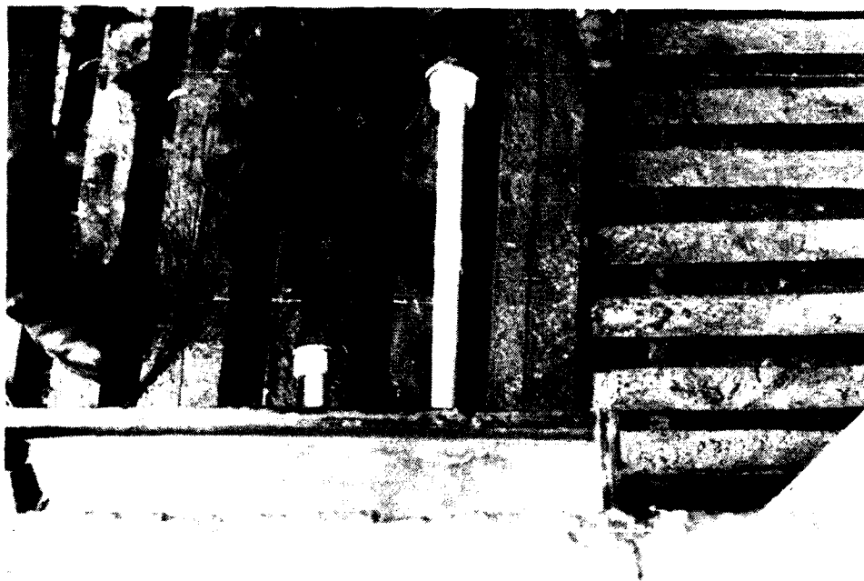
a. Anchor being spun into a submerged hole
