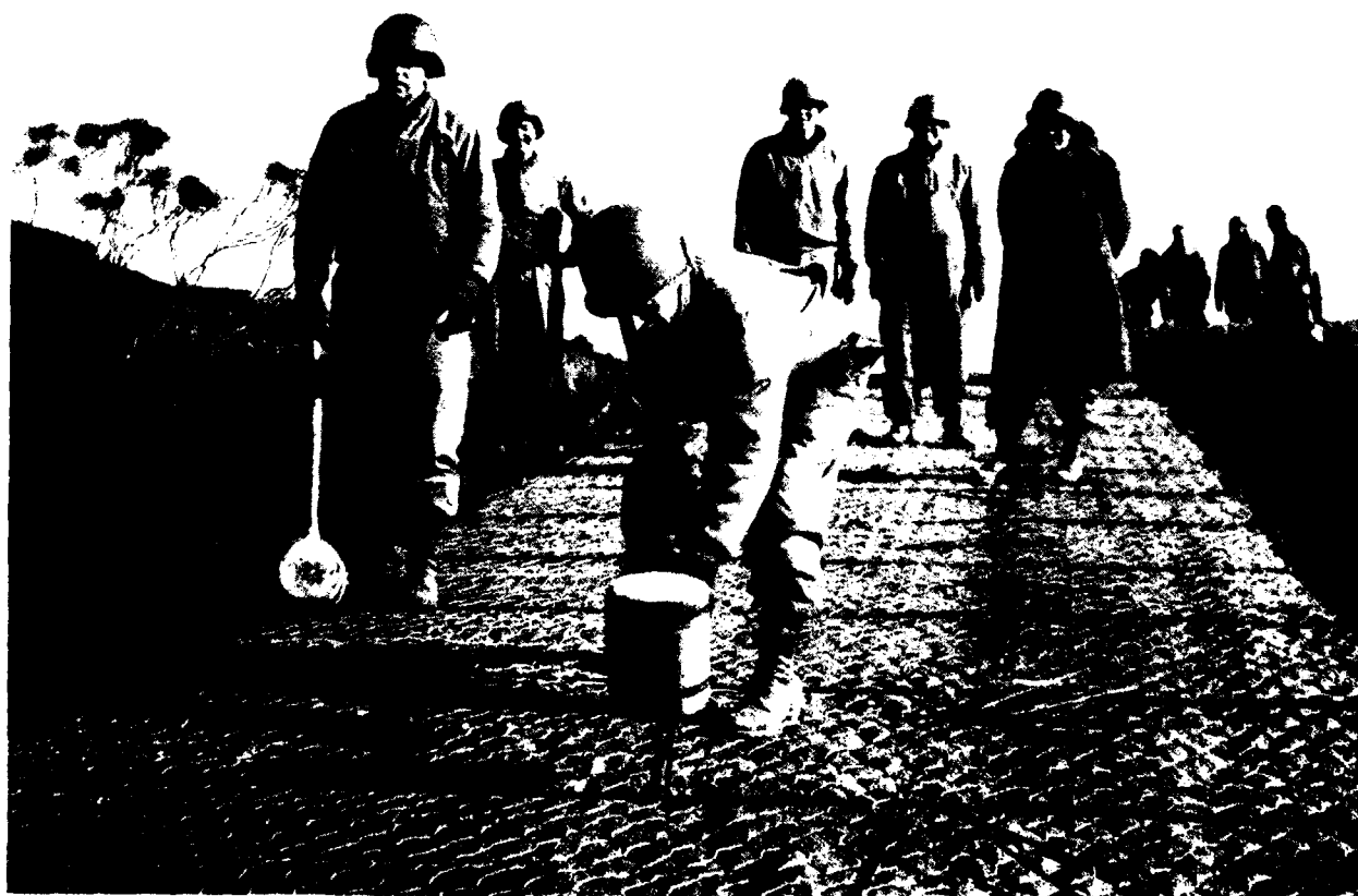
PUTTING DOWN ROAD MATTING at the beach exits was one of the problems confronting the engineers after the landings. Many heavy vehicles and the rapid supply build-up made the construction of a number of such roadways necessary.
