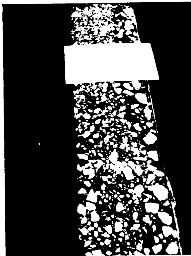
Photo 6. Cross section - Slab 1
