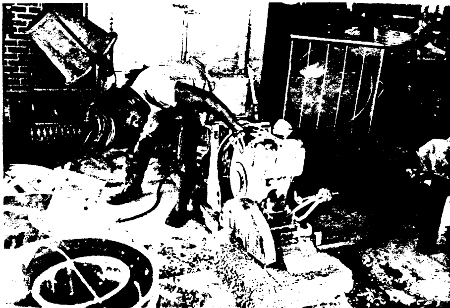
Figure 3.5 Concrete Sawing PMA Specimens into 6-in. x 6-in. x 20-in. Sections.
