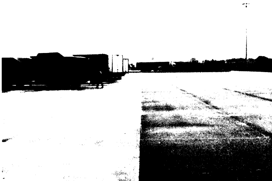
Photo 1. Commercial parking facility - Niort, France
