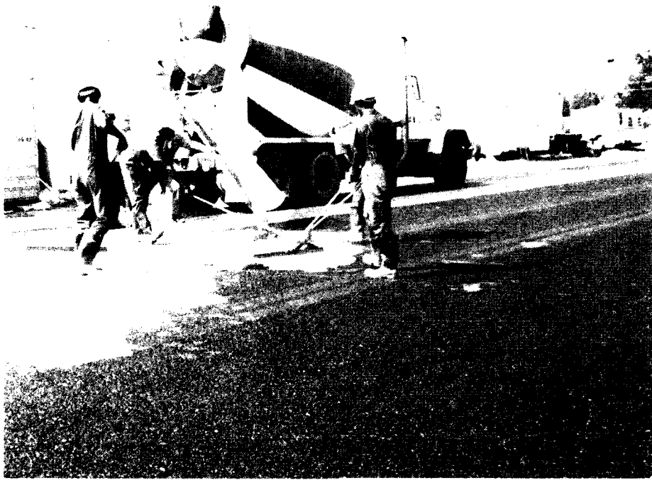
Figure 9. Resin modified slurry grout being applied to open-graded asphalt mixture
