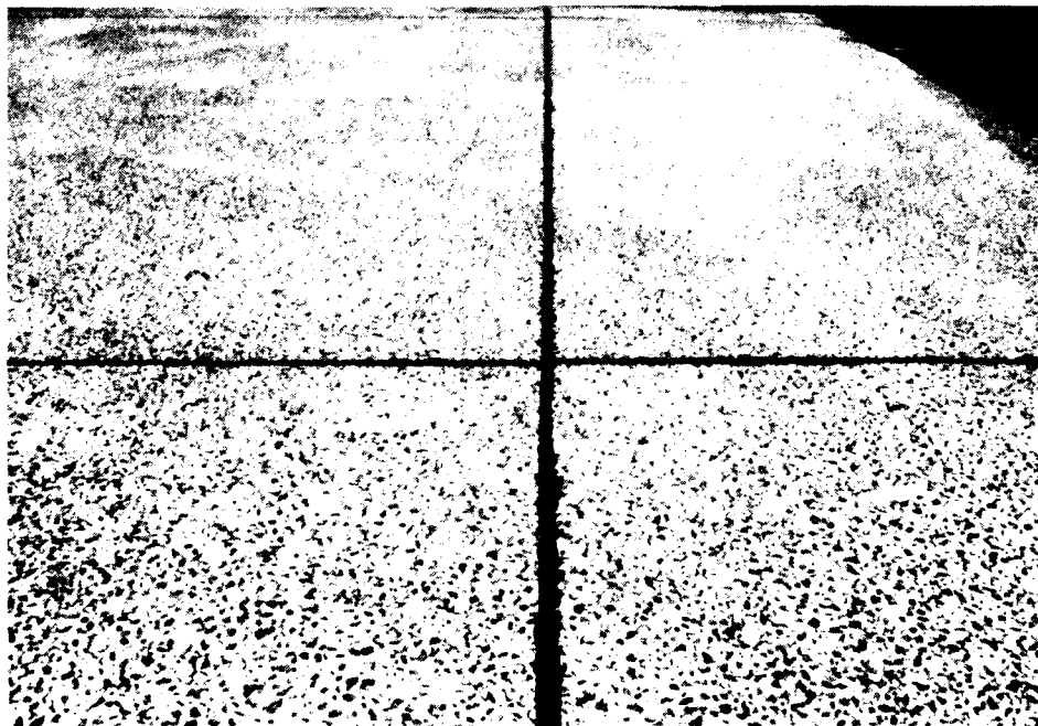
Photo 6. Typical condition of sawed joint in 1979 Salviacim pavement
