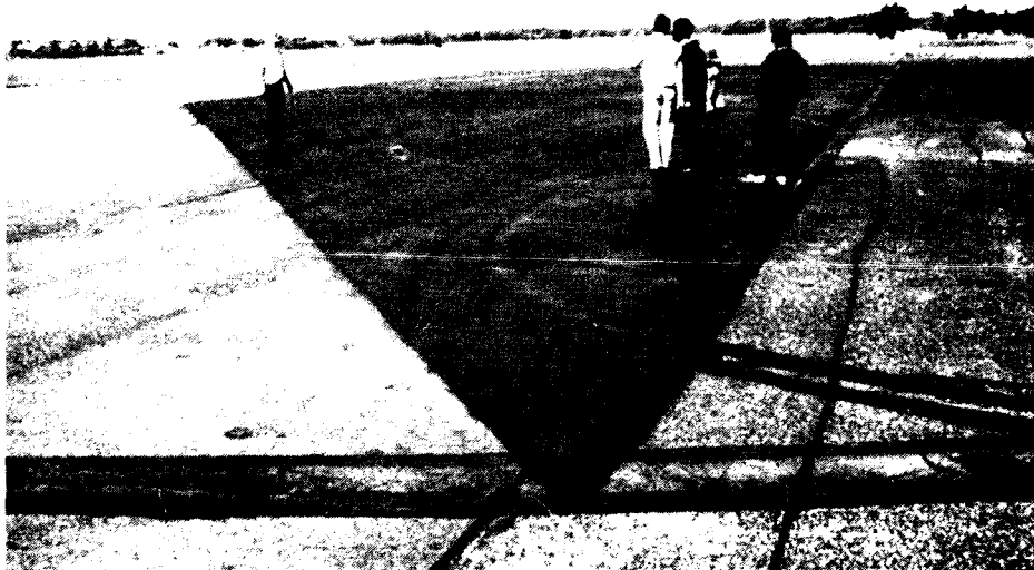
Photo 11. Asphalt concrete pavement that was sealed with Promak
