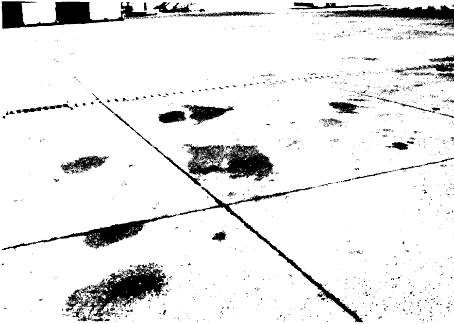
Photo 9. Jet fuel spillage on parking apron
