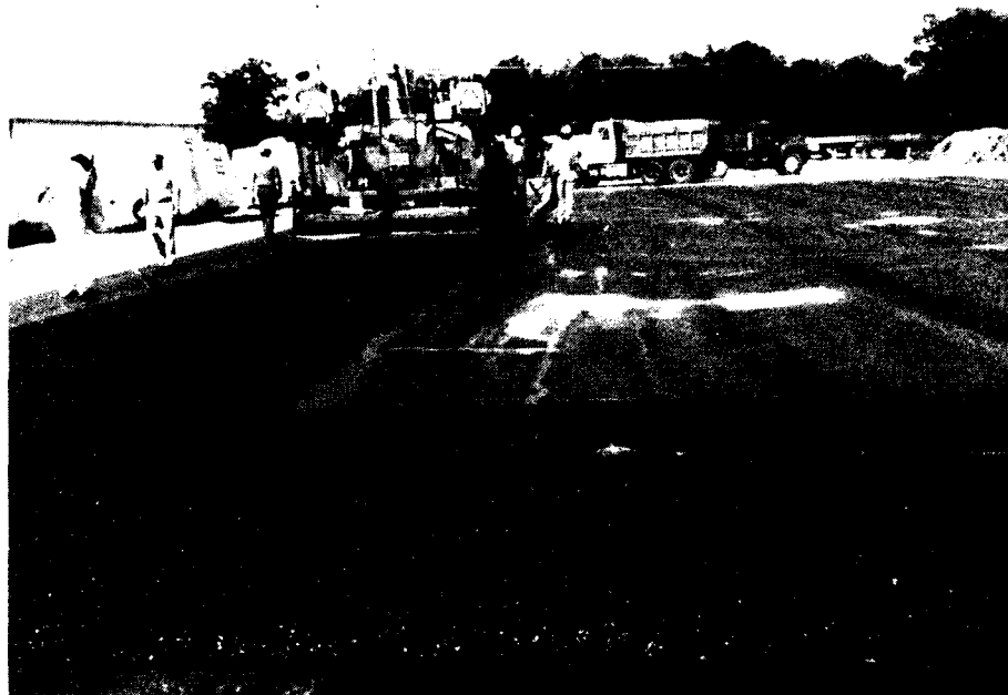
Figure 6. Placing open-graded asphalt material
