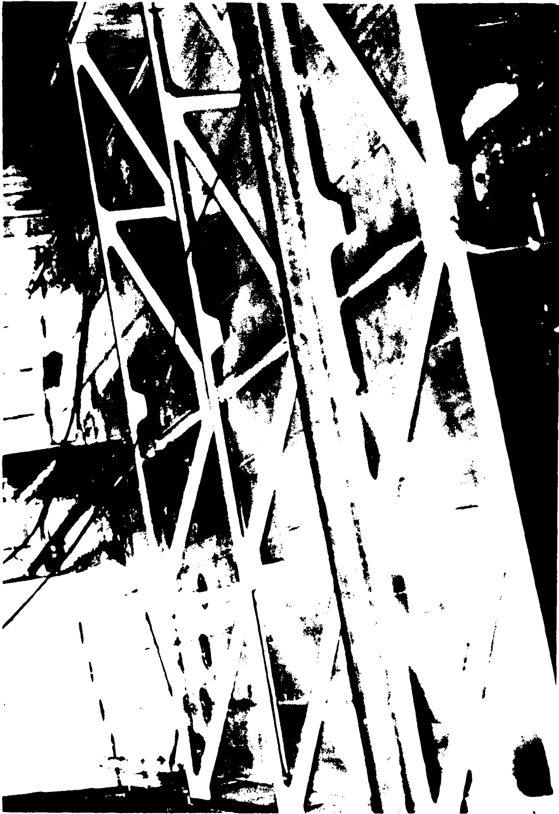
Figure 6. Installation of Internal Trusses
