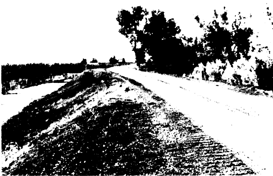
Figure 7. General view of levee at study site showing vegetation growing on riverward side and burned-over slope on landward side
