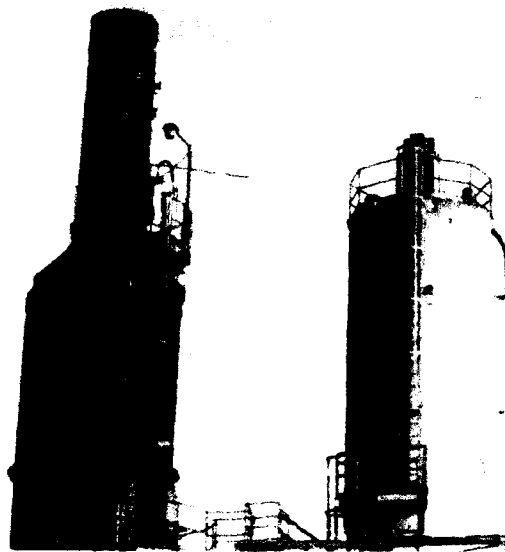
Figure 19. Rainout deposits on scrubber shell and adjacent lime silo.
