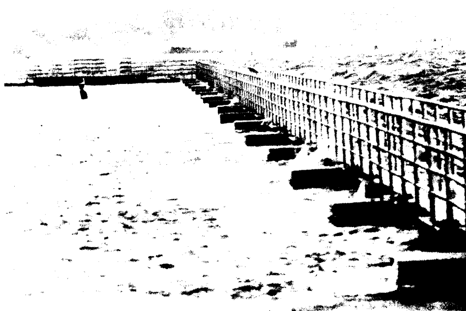
d. View of shoreward leg showing relatively calm inside conditions despite overtopping
