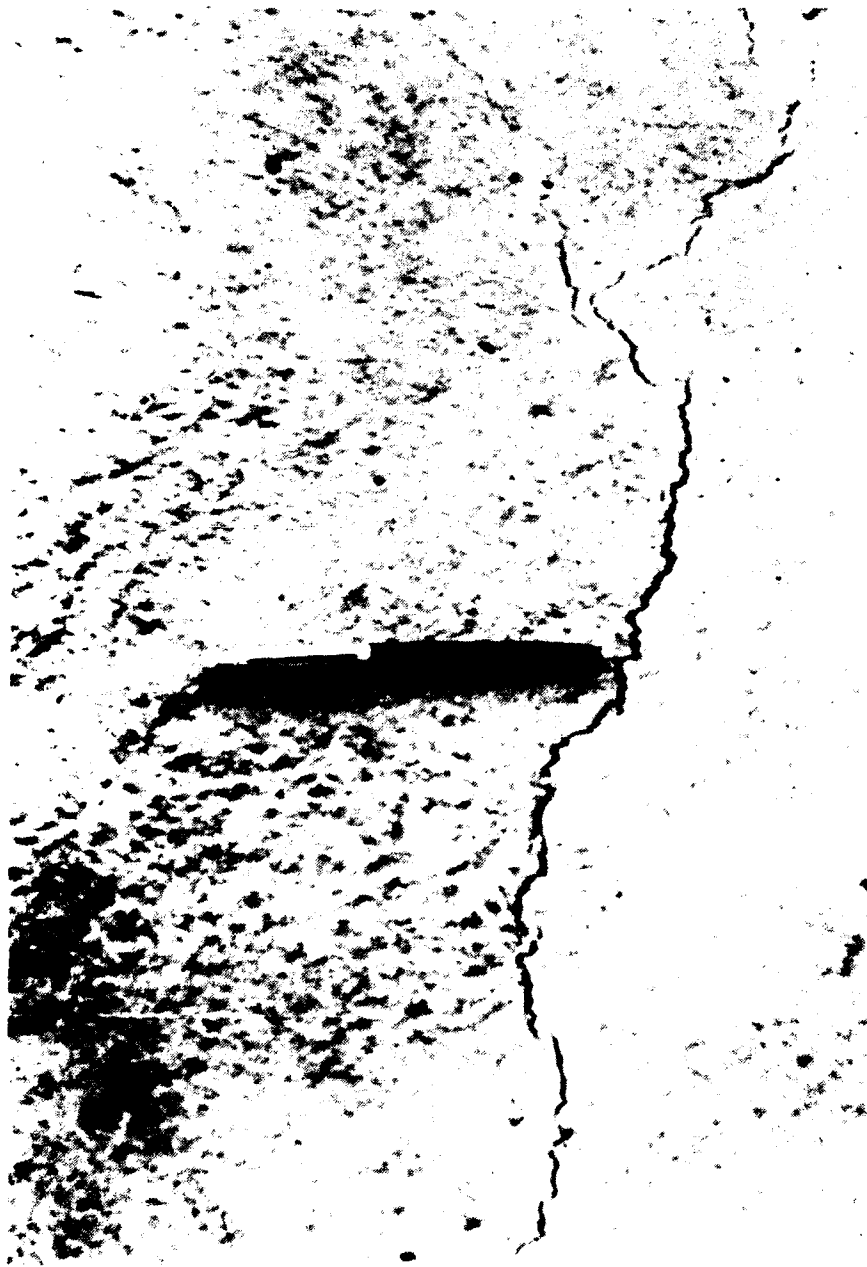
Figure 18. Plastic shrinkage crack.
