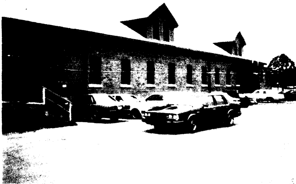
Figure 5. Building 17, south rear view.
