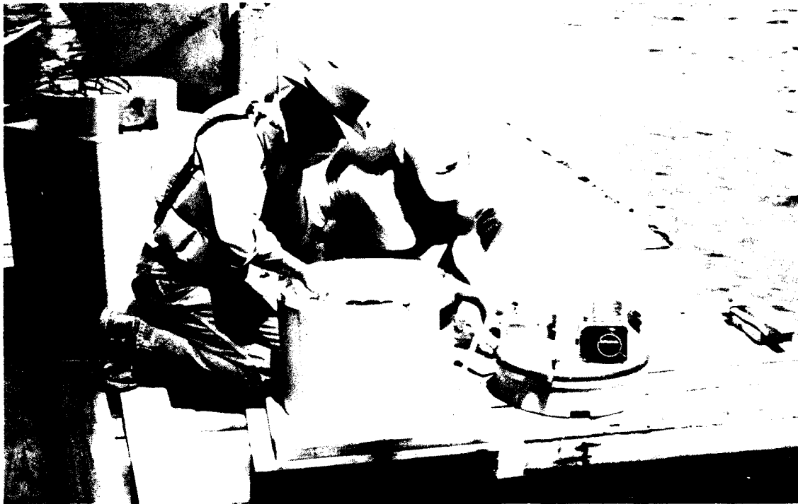
Figure 4. Field installation of water sampler
