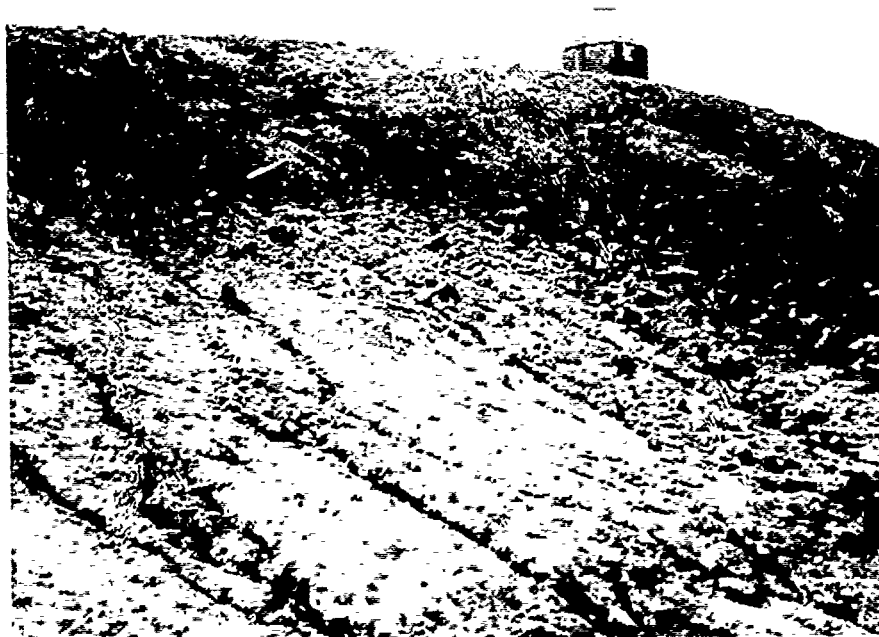
Figure 8. Erosion on a recently renovated igloo.
