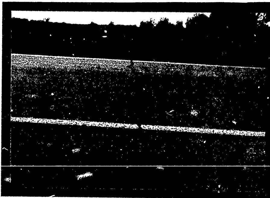
PHOTO 19: EVENLY SPACED SHRINKAGE CRACKS SUCH AS THESE ON TAXIWAY F ARE UP TO HALF AN INCH WIDE AND SHOULD BE ROUTED AND SEALED ASAP (TYPICAL).
