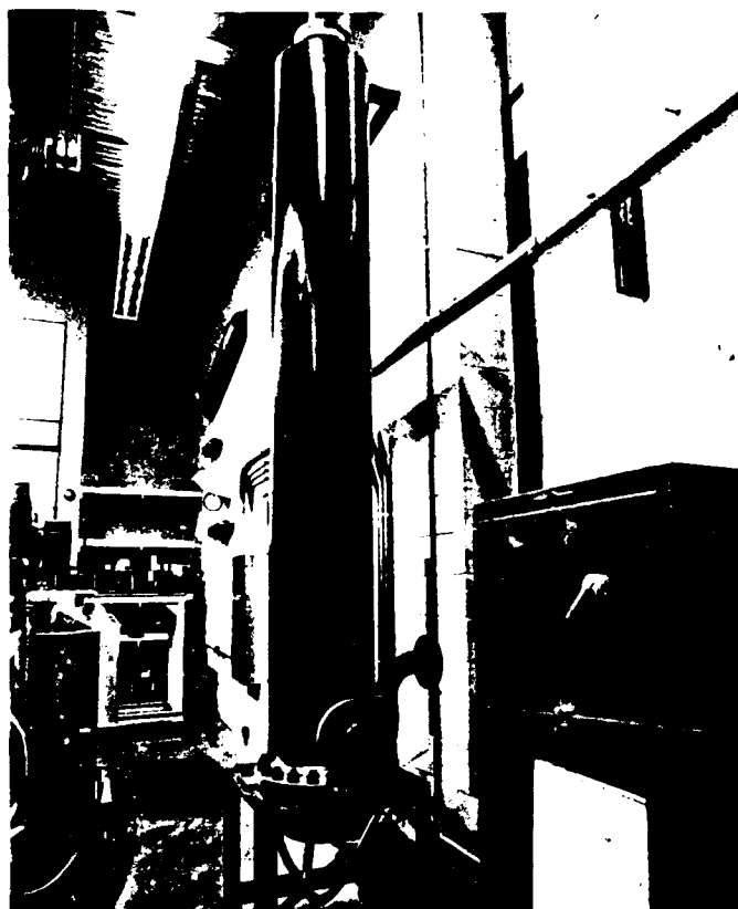
b. Air Heater Mounted on Wall
