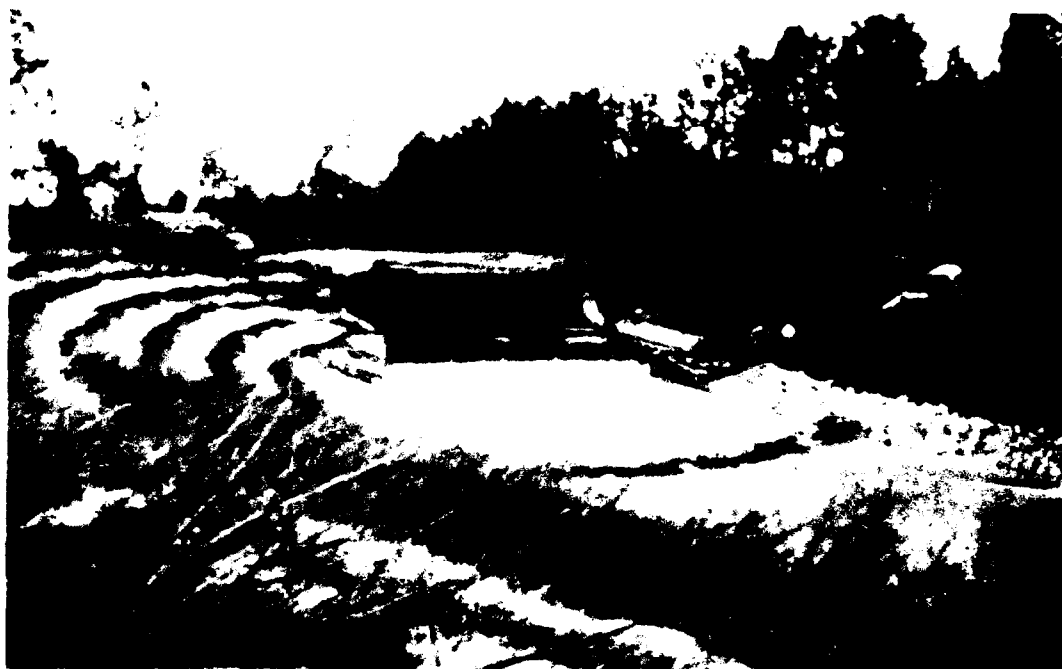
Photo 3. The existing drop structure in the final stages of construction activities. Note the soil bioengineering brushlayers on the left.
